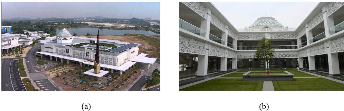
Figure 1. Modern mosque in Cyberjaya with passive cooling and lighting strategies; (a) double glazing glass dome at roof level and (b) central courtyard for cross ventilation and daylighting.
