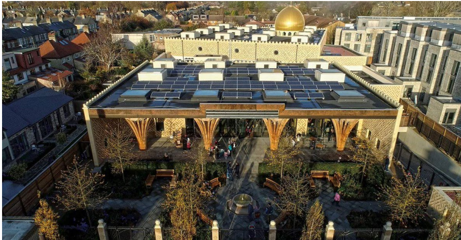
Figure 4. A British mosque for the 21 st century with an environmental design principle that includes a skylight and solar PV on the roof.
