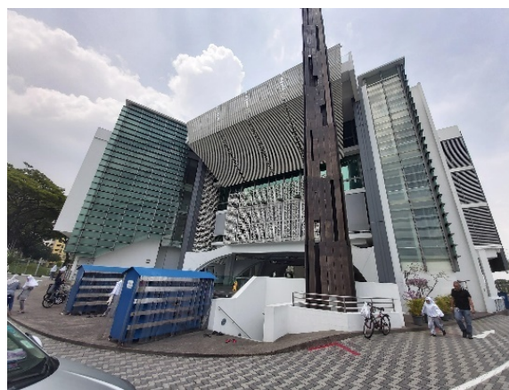
Figure 6. The main entrance of the mosque (facing east/opposite kiblat)
