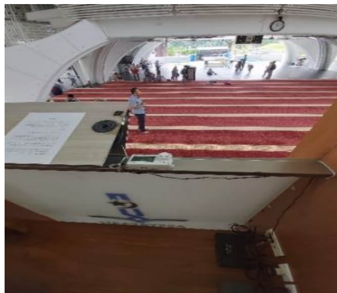
Figure 12. View from mimbar towards the main entrance; entryway connects to the main prayer hall without any wall constructions allows for free airflow movement.
