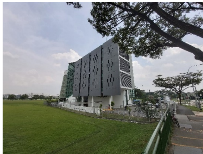
Figure 10. Southside of the building
