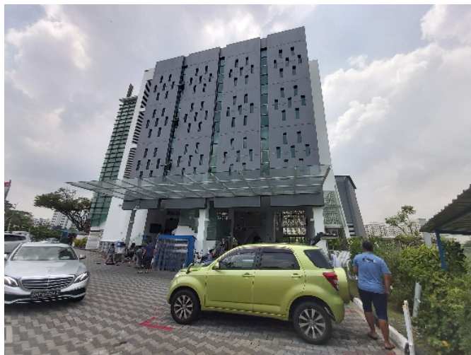
Figure 7. Side entrance of the mosque (facing north)
