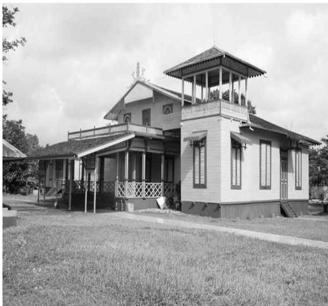
Figure 25. – The Matan Palace in 2010, after renovation. Collections include thrones, furniture, batik and other textiles, and portraits and photos. (Source: http://liveinbalikpapan.blogspot.fr/2012/09/kerajaan-tanjungpura.html ).
