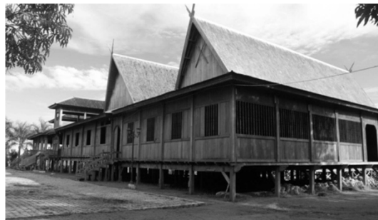
Figure 19. – The Istana Kuning, after renovation. The three main buildings, and the entrance and tower in the background. (Source: http://aditya-pbun.blogspot.fr/2013/07/kesultanan-islam-pertama-di-kalimantan.html ).
