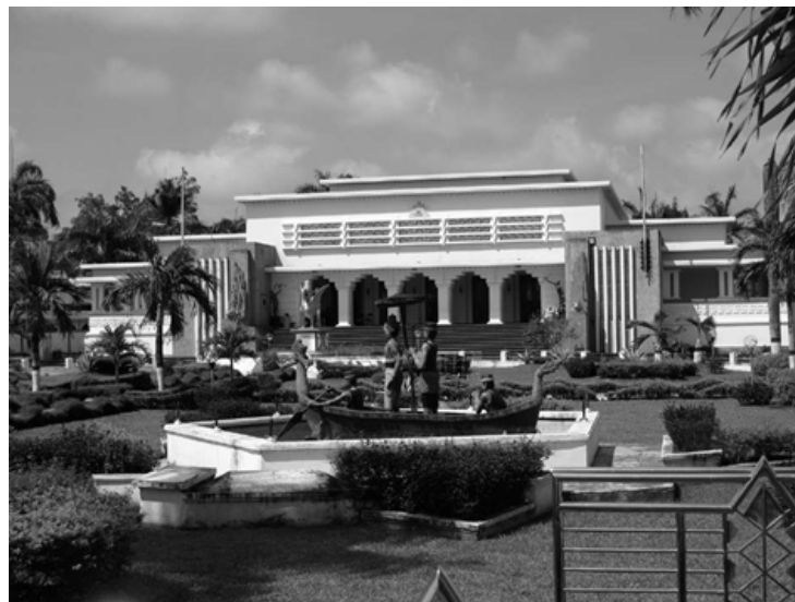
Figure 6. – The “colonial” Kutai Palace, built in concrete by a Dutch architect for young Sultan Aji Muhammad Parikesit at Tenggarong. Decorated in Art Nouveau style, it faces the Mahakam River across vast front grounds. Started in 1932, it was handed over to the sultan in 1936. After the abolition of the sultanate (1960), the palace was turned into a museum by the military commander of East Kalimantan (1971), then became a state museum, Museum Negeri Mulawarman, in 1979. The obelisk disappeared, but all sorts of fancy new monuments appeared on the front grounds, including a large replica of the winged Lembu Swana, the kingdom’s symbol. The museum houses royal paraphernalia, court costumes, archaeological objects, historical documents, a large collection of ceramics, and an ethnographic section of Dayak artefacts (Photo: Bernard Sellato, 2010).
