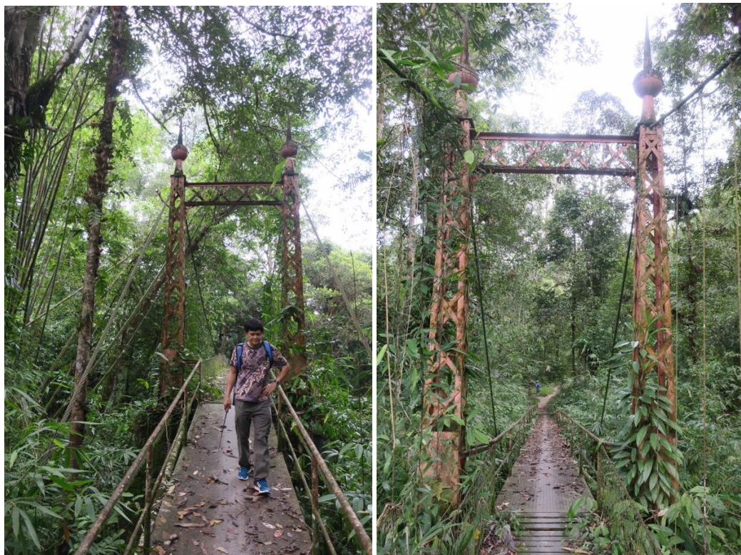
Fig 3. The Red bridge in Seropak 2018 (Photo Ib Larsen)
