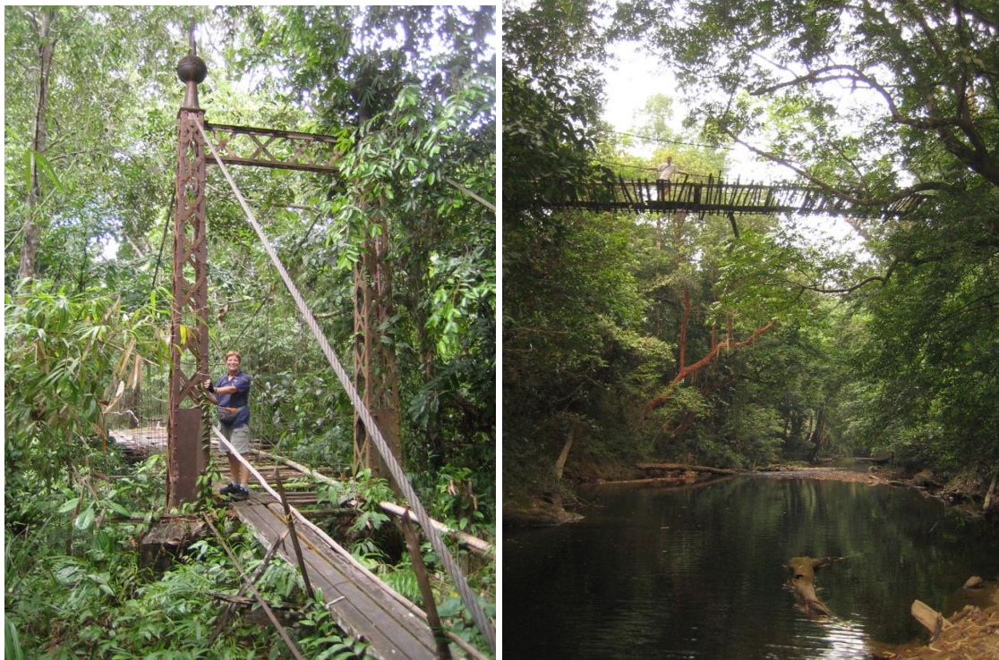
Fig 1. The Red Bridge in Seropak July 2005 (Photo Ib Larsen)
